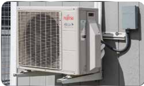
MINI SPLIT HEATER/AC UNIT 12,000 BTU Unit Requires 110-V A-C 24,000 BTU Unit Requires 220-V A-C Low Temp Units Available for Colder Climates
