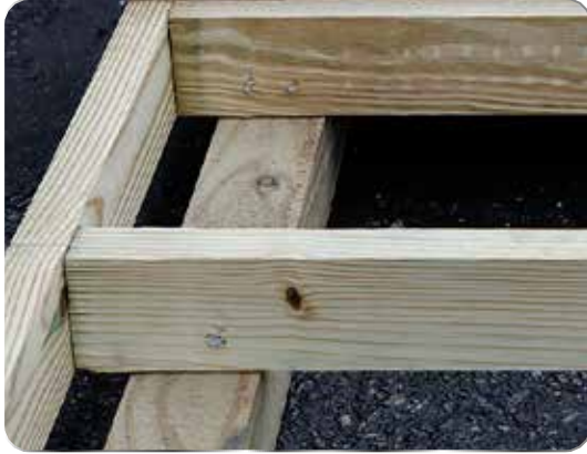
Pressure Treated 2x4 Floor Joists 4x6 Runners
