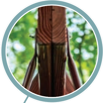
Heavy-duty, double 2x6, vertical-edge swing beams.
